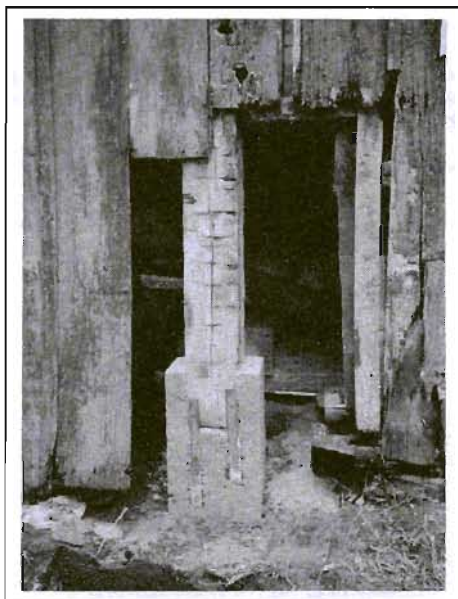
Concrete and steel braces strengthen post in barn.
