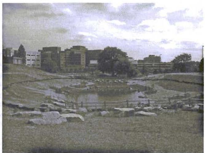
The stormwater detention system was built in the summer of 2004 and is located between the Art and Architecture building and the Engineering Research buildings on North Campus. Stormwater from the central area of the campus flows into the detention system, which consists of three cells. The cell system slows down the flow of water, modifies its temperature, and allows particulate matter to settle out. Eventually, the water slowly flows to the Huron River.
