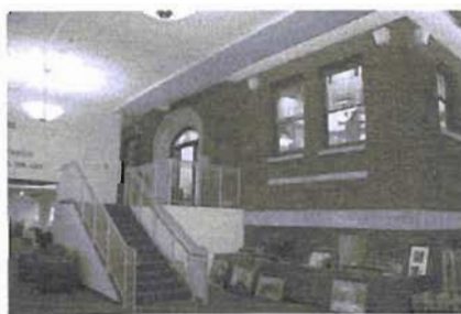
Angola, IN – original building enclosed in the new addition
