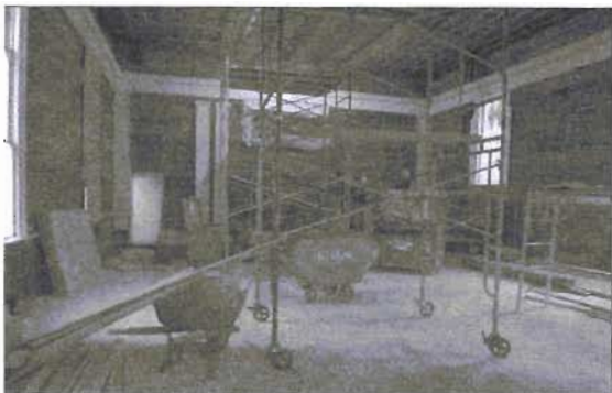
Wide-board interior sheathing visible after removal of plaster
