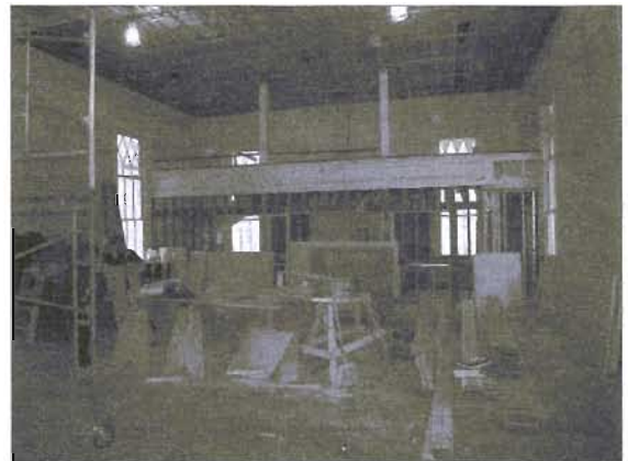
Demolition of narthex area
