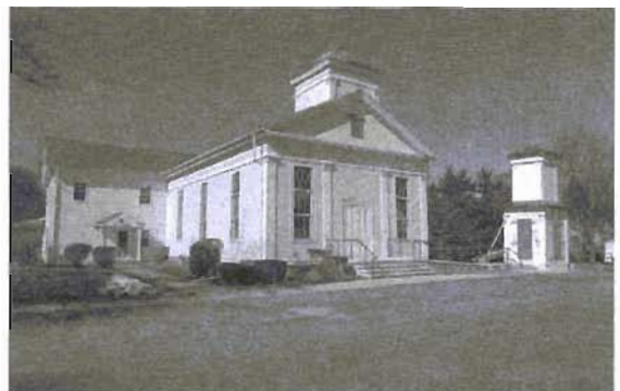
Church with finished steeple waiting to be raised
