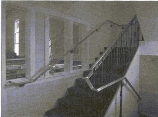
New modern stairs to balcony
