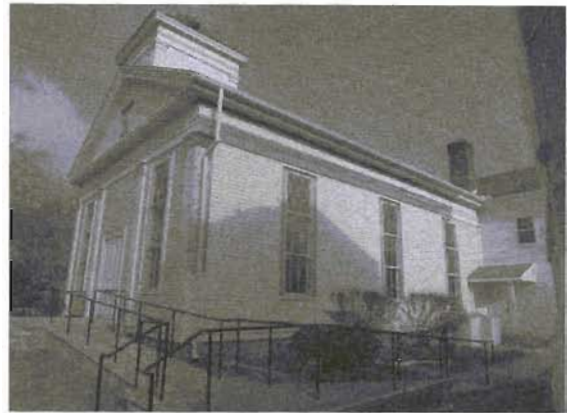
Exterior of church showing new ramp and railings
