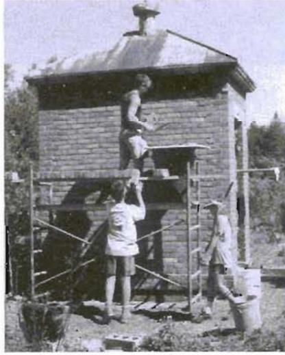
The brick oil house was vandalized and many of the bricks were stolen. In 1991, the scouts of Troop 4 replaced the missing bricks which were difficult to find because of their irregular size.
