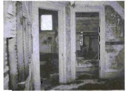
The photo at the right shows the condition of the keeper's quarters in the mid-1980s. Fortunately, most of the door and window trim were relatively intact.
