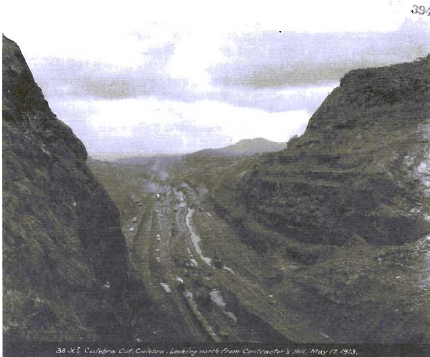
38-X2 Culaybra Cut, Culabra, Looking north from Contractor's Hill, May 17, 1913.
