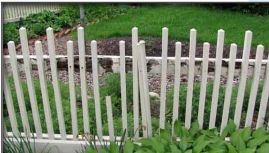
**BEFORE:** Broken spindles, rotting wood
